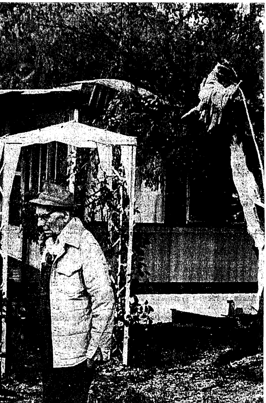
The Wednesday storm of last week knocked this part of a locust tree over on the roof of the M. N. Benjamin home in Juliaetta, causing severe damage to the structure. Mr. Benjamin's home was just one of
