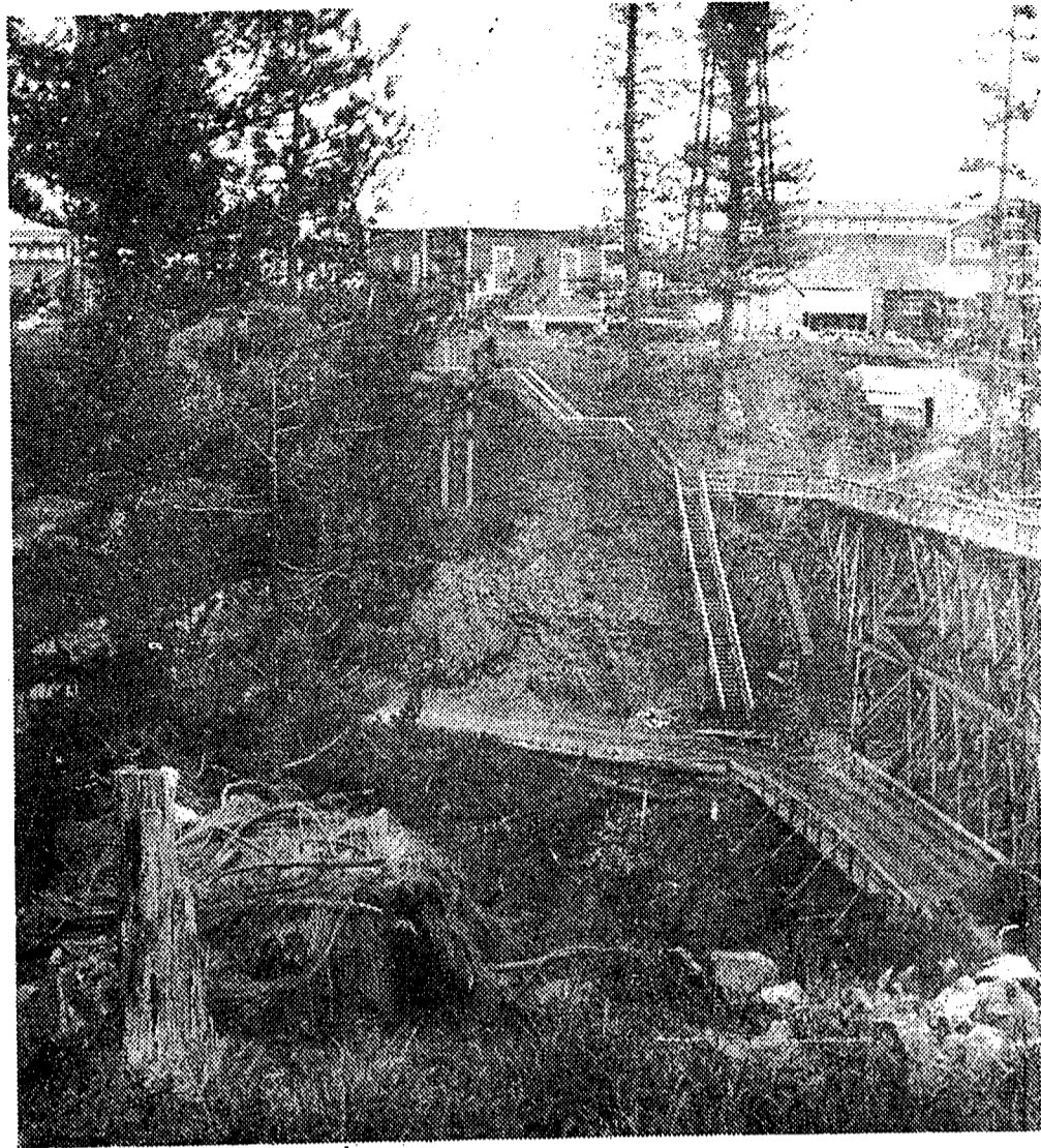
The old Winchester mill and foot bridge with U. S. 95 in
