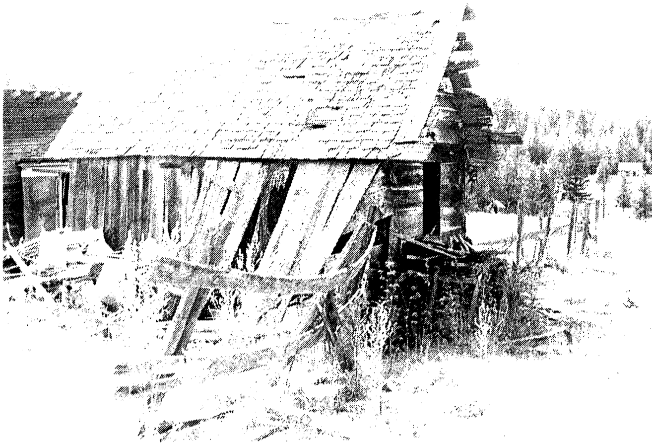
Wind and weather have taken their toll on this shed still standing on an abandoned homestead near Westlake.
