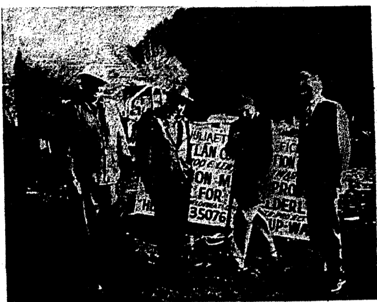
FIRST SHOVEL TURNED—Mayor Harold Freeman of Juliaetta turns the first shovel of earth to mark the beginning of the Johnson Manor Apartments. Others looking on from left to right are Neal Knightland,
