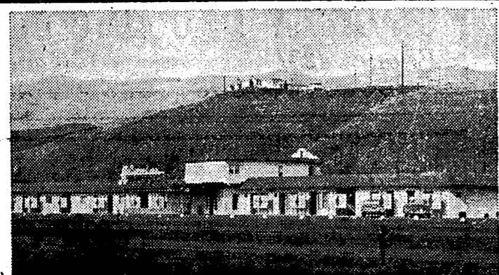
THE HOLLYWOOD INN, 3001 N. & S. Highway, Lewiston, "Electric Heat has proven a wise choice for our Motel because it's so easy to maintain and operate, and the space we save adds to our rentable income," said Mr. E. J. Klumper, Owner.
