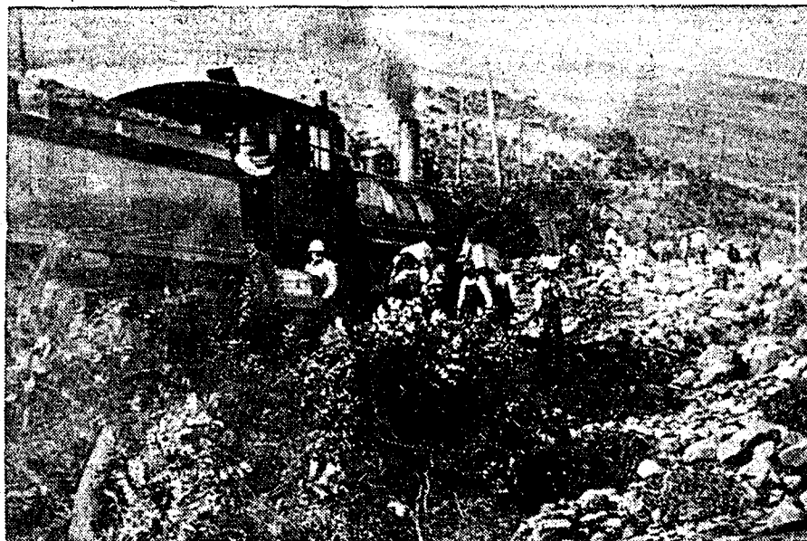
The Spokane-Lewiston train stopped by a washout 3/4 miles east of Jullaetta in 1912. Note men carrying boxes and luggage from the stalled train to another the other side of washout. Other train not shown.
