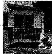
JACKED-UP HALF is lowered onto foundation footings laid earlier. Homes have 680 square feet of living space, sell for \$6,990 each within a 500-mile radius of Leesburg plant. Price includes hauling of six-ton halves and cost of foundation.
