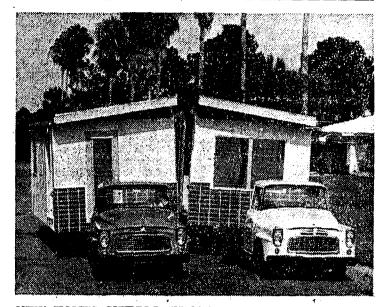
NEW HOMES SHIPPED IN TWO PIECES is prefabricating twist that a Leesburg, Fla., construction firm has recently developed. Idea allows buyers to occupy their new two-bedroom dwellings a mere 12 manhours after its halves arrive by Inter-national truck at building site. Even cabinets and wiring already are in place. All that remains to be done is bolt halves to each other and to foundation.
