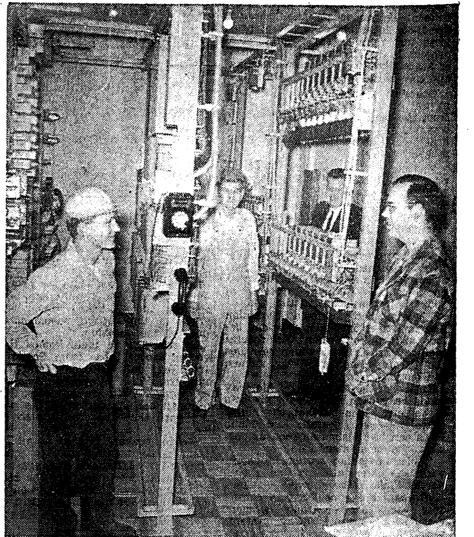
POTLATCH TELEPHONE CO. INSTALLS DIALS
