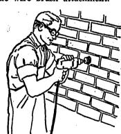
Portable drill fitted with wire brush cleans masonry quickly.
