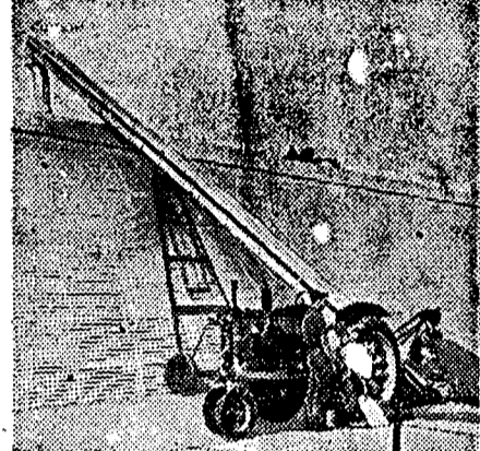
Grain being loaded into Quonset huts for CCC storage near Paulding, Ohio.
