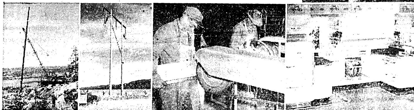
Through forests and across mountain torrents, lines are pushed forward, to bring low-cost Cabinet Gorge "Reddy" kilowatts to homes, farms, and industries throughout the Inland Empire.
