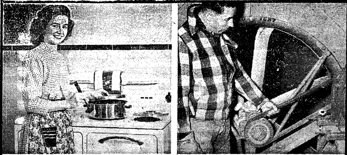
Farm life in the Inland Empire is more pleasant and profitable now that low-cost electricity is available to nearly all farms. The beautiful electric kitchen at the left and the efficient hay-drier at the right are just two examples of many ways electricity is used for better farm living and better farming.
