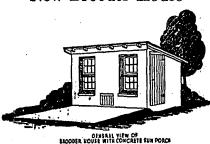
A stationary concrete brooder house and sanitary sun porch, as shown, provide maximum protection for chicks. Disease problems become greatly reduced when concrete sun porches are provided. The concrete is also a safeguard against fire in the brooder house.
