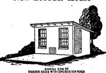
A stationary concrete brooder house and sanitary sun porch, as shown, provide maximum protection for chicks. Disease problems become greatly reduced when concrete sun porches are provided. The concrete is also a safeguard against fire in the brooder house.
