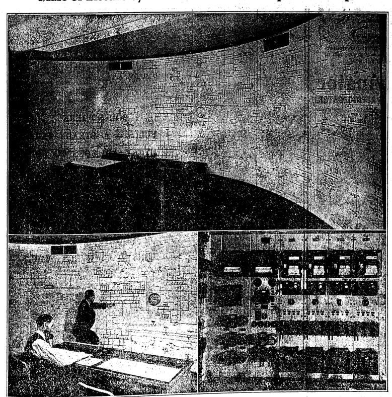
A complete picture of the Washington Water Power company's electric system is provided the system operator on the power board shown at the top. The plan is a miniature, enabling the system operator to provide an immediate service for maintenance of power over the network of lines between the Cascades and Rocky mountains. At the lower left Engineer M. L. Blair is to be seen at the power board, while Ray L. Wetherell, system operator, is hand-
