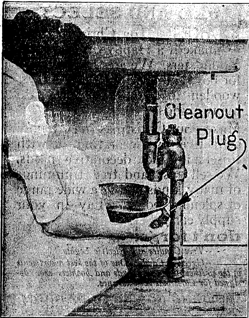
Cleaning Out a Sink Trap.
