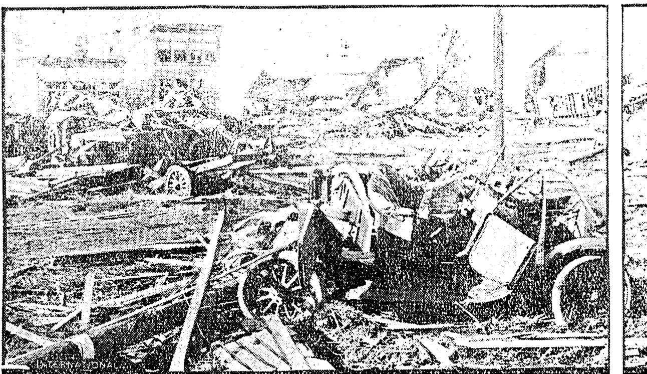
View of the business district of the town of Davis, S. D., which was totally ruined by the recent severe tornado which swept South Dakota.
