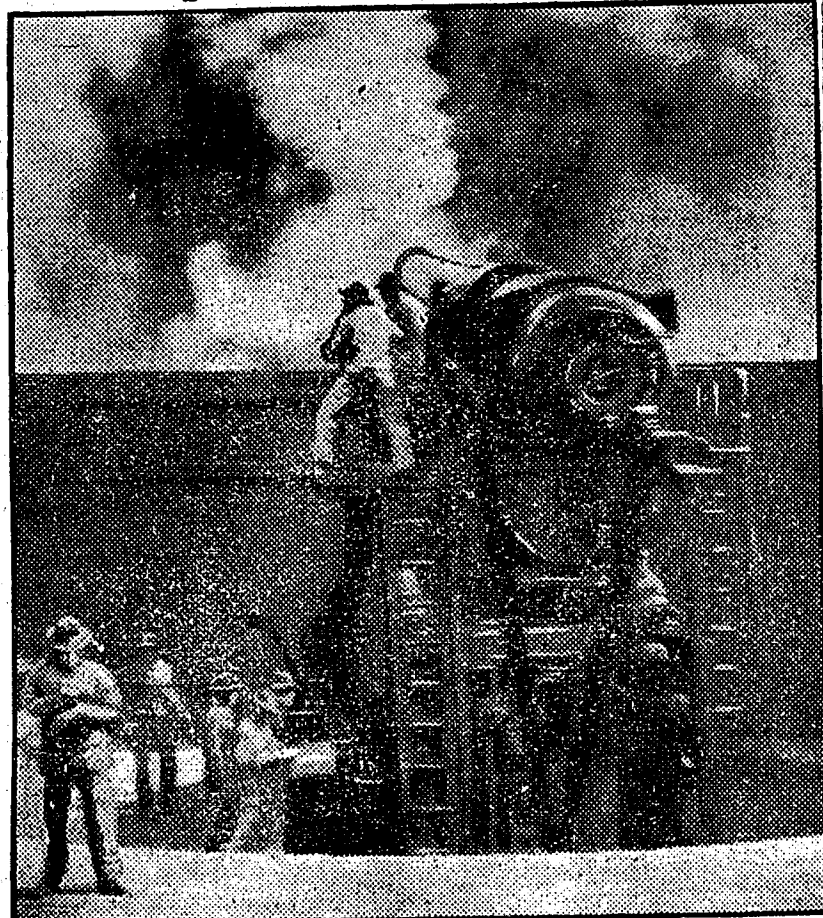
THIS is a 12-inch coast defense gun in action at Fortress Monroe. The weapon is of the disappearing pattern. It pops up "over the top," bangs away and vanishes—so far as the foe can see. It is the most powerful gun of its type.
