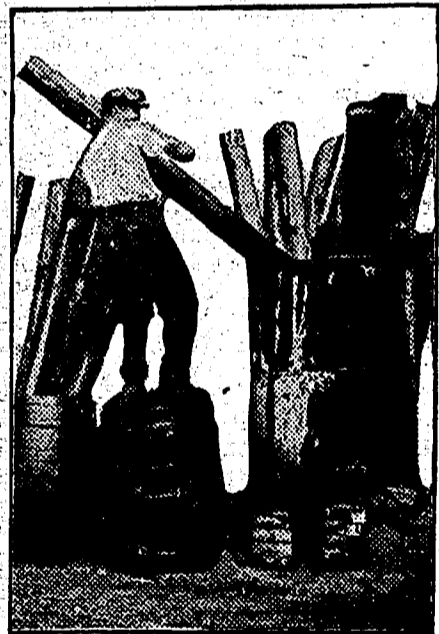
Removing Posts After Treatment in Creosote—The Posts Are Allowed to Drain in the Barrels.
