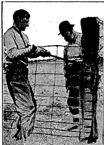
Attaching the Wire After it Has Been Stretched.
