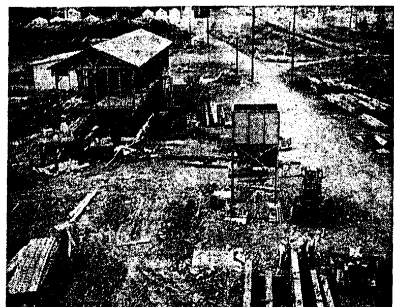
The new mill itself, showing the chipper (left center); chip surge bin (center) and the saw mill building with filing room on the left. (Photos courtesy D. H. Jones)
